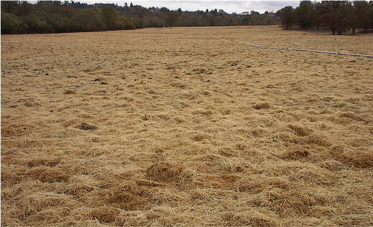
The most effective erosion control practice (both in terms of protection and cost) is the use of cover crop and straw mulch. Straw provides a cushion between the disturbed soil and the velocity of the raindrop. It's the best insurance for **protection** from the early rains if you cannot plant your cover crop in mid-September and irrigate it.
